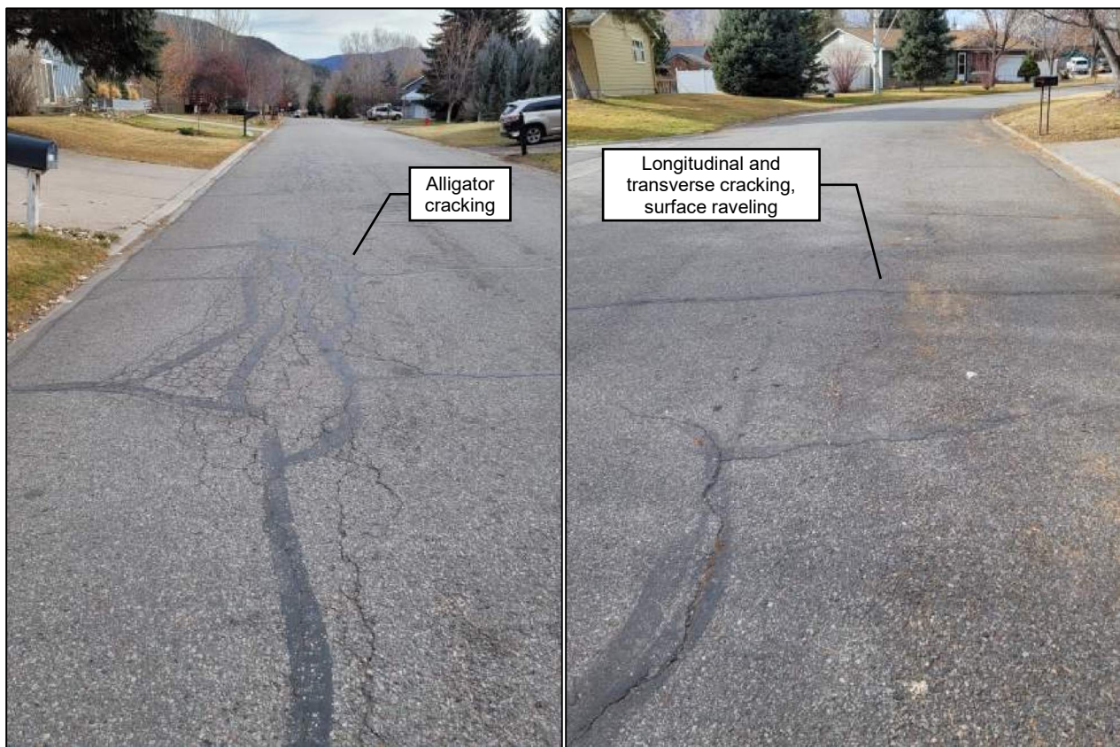
Figure 3-4. Cheyenne Roadway Conditions
