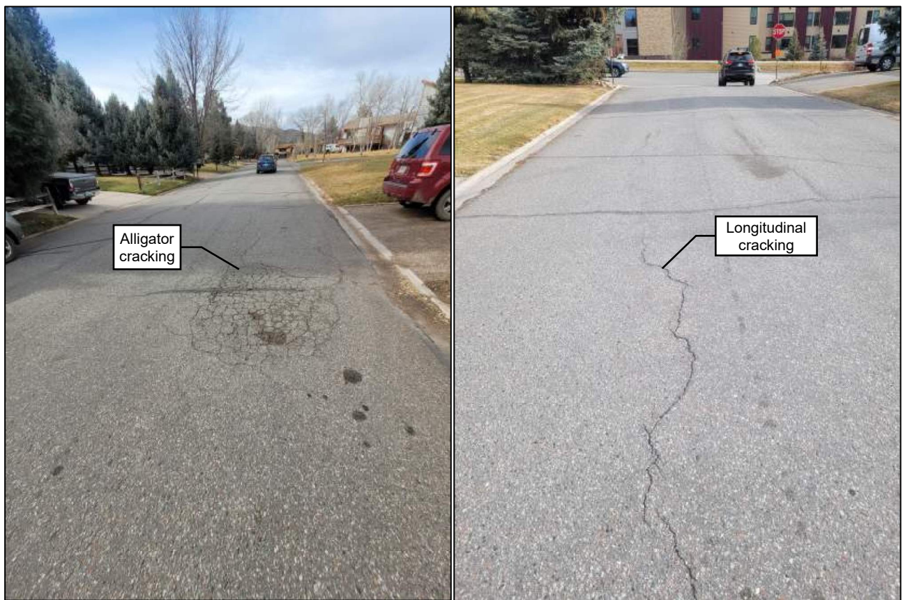
Figure 3-10. Hopi Roadway Conditions
